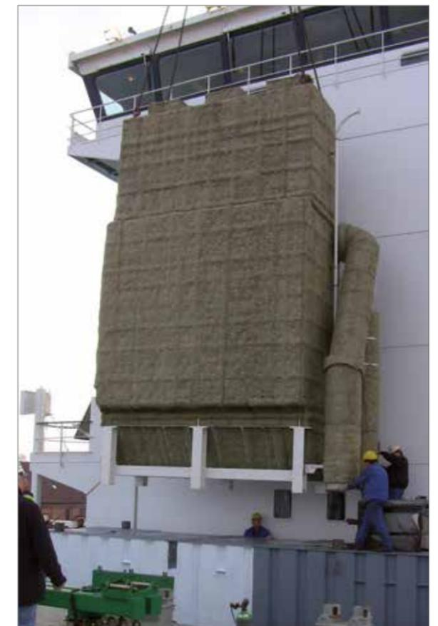
**Figure 51: Installation of a Couple Systems dry exhaust gas cleaning unit**
