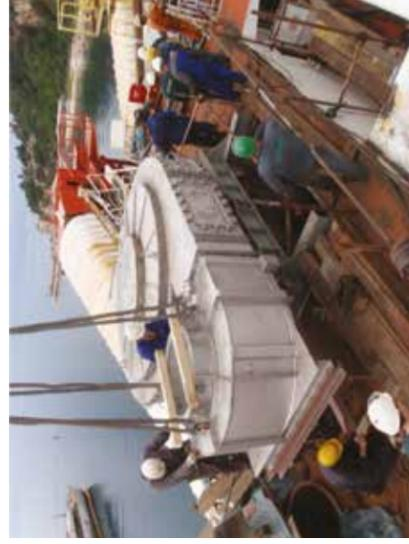
New fan housing and lower part of funnel, installation of outer pipe, installation of inner pipe, installation of upper part and bypass lines
