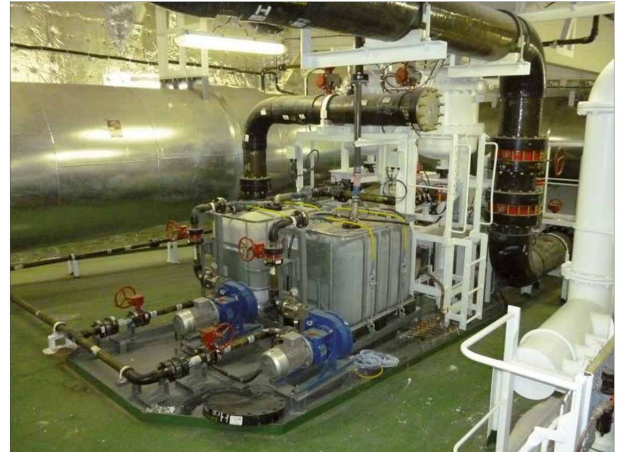
Figure 47: Washwater treatment residue collection
