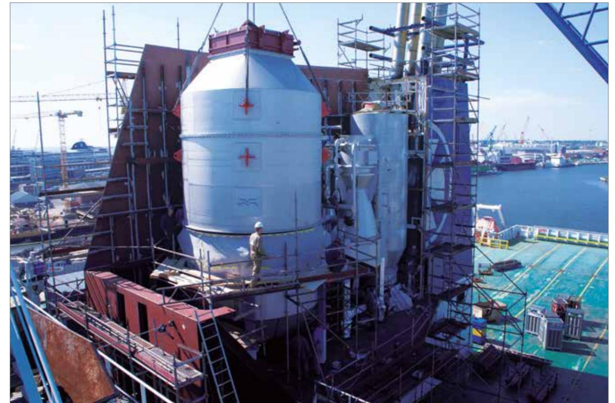
Figure 41: Alfa Laval's trial EGC unit during installation
