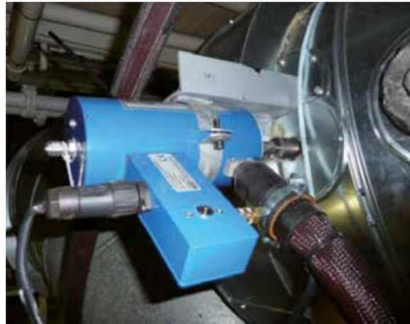
**Figure 44:** Heated sample line and probe for extractive analyser
