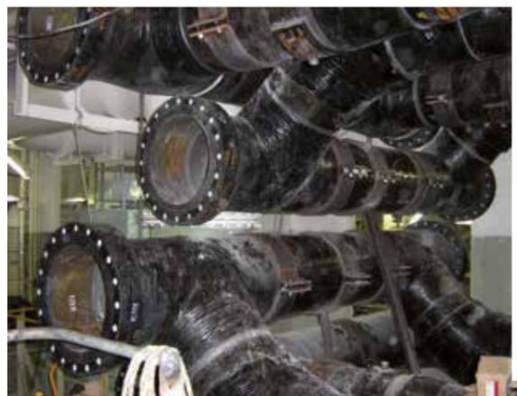
Figure 27: Glass reinforced epoxy pipe construction
